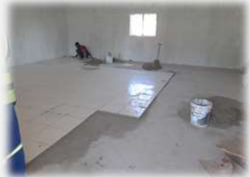
Tiles have now been laid in all rooms
