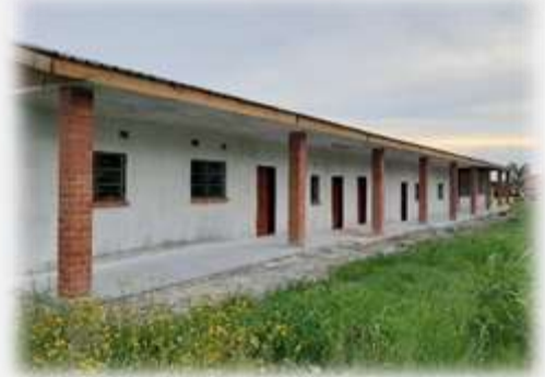
Terrazzo laid on the veranda, doors fitted and builders off sight
