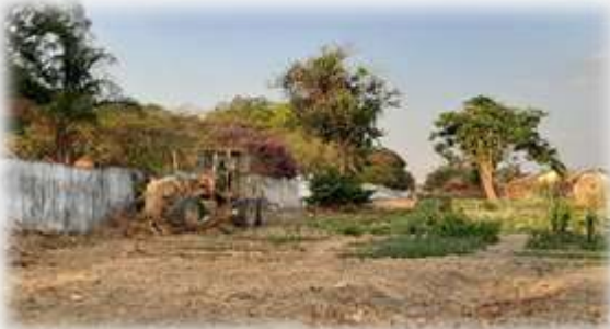
Clearing grass and levelling the ground
