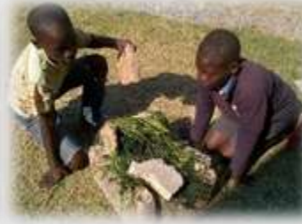
Building houses using natural materials
