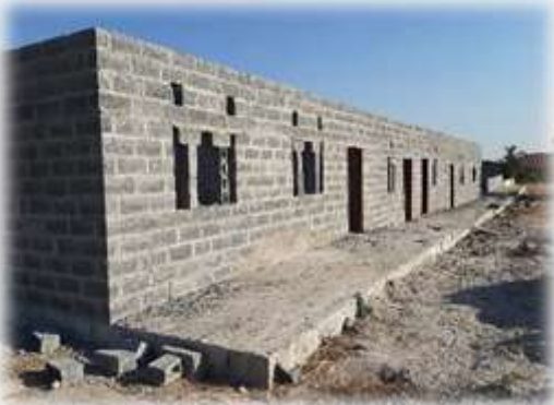
Arise block walls completed.
