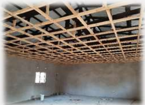
Arise block ceilings in place
