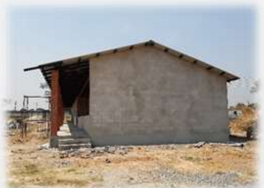
Arise block plastered, ready for painting
