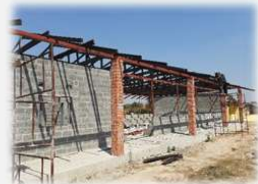
Arise block roof in place in the dry season
