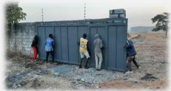
Lifting our new gate into place
