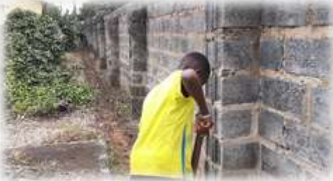
A number of our pupils had piecework digging trenches for cables
