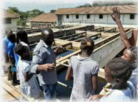
Visiting the water treatment works
